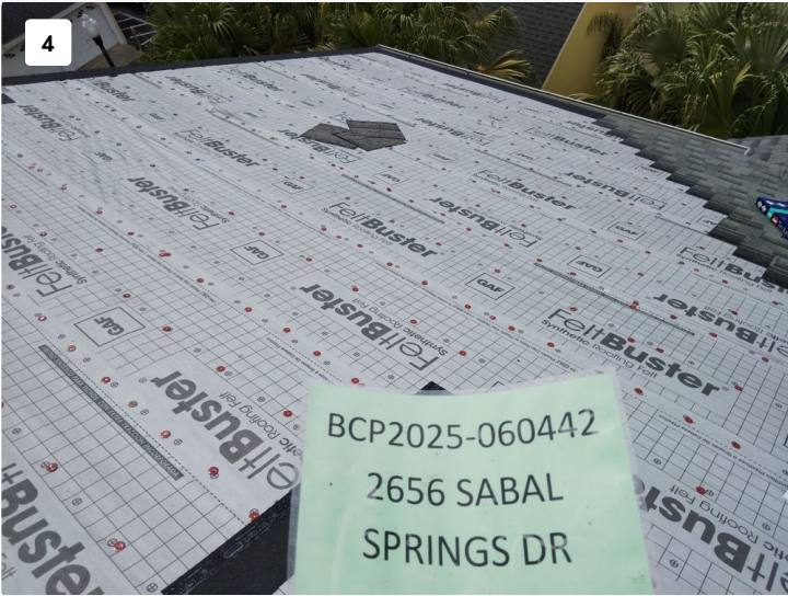
Project: 2656 Sabal Springs Dr Date: Jun 19, 2025, 4:36 PM Creator: Lucio Roofer
